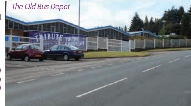
Building 5 Vantage Point Business Village from Bradley Court Road
