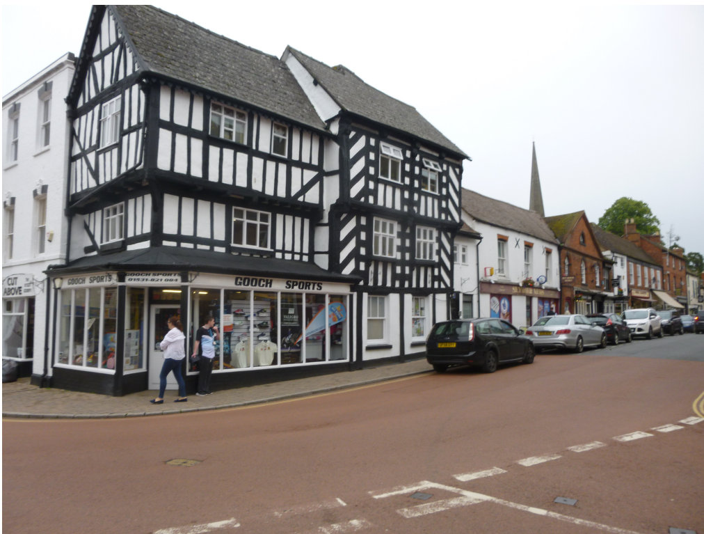
A Grade II* listed building in the foreground
