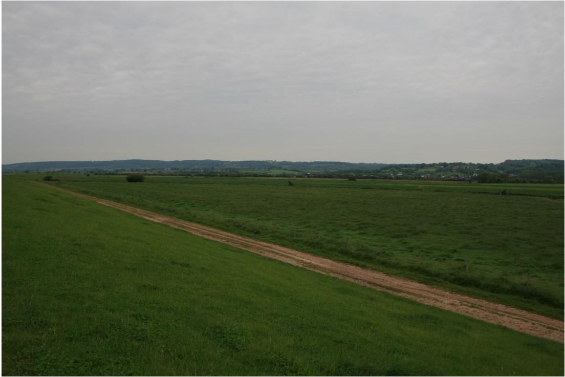
Photograph 7 - View across the Lydney New Grounds from the top of the inner embankment
