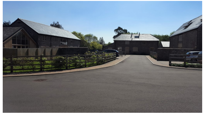
Duncastle Court—Barn Conversions
