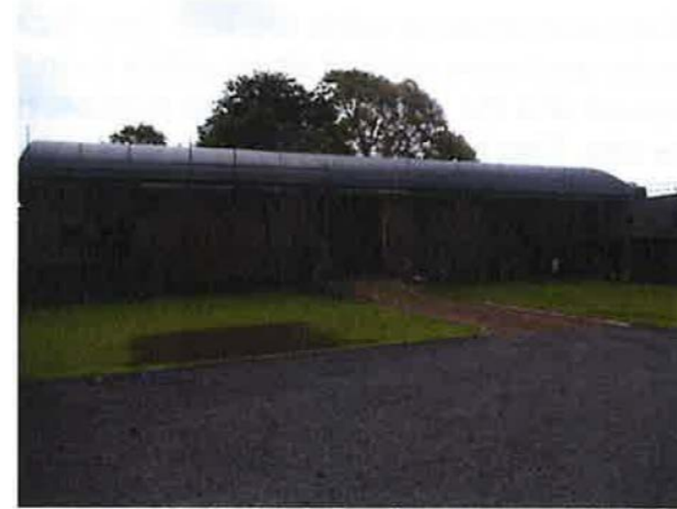
Main barn slow repair 2017
