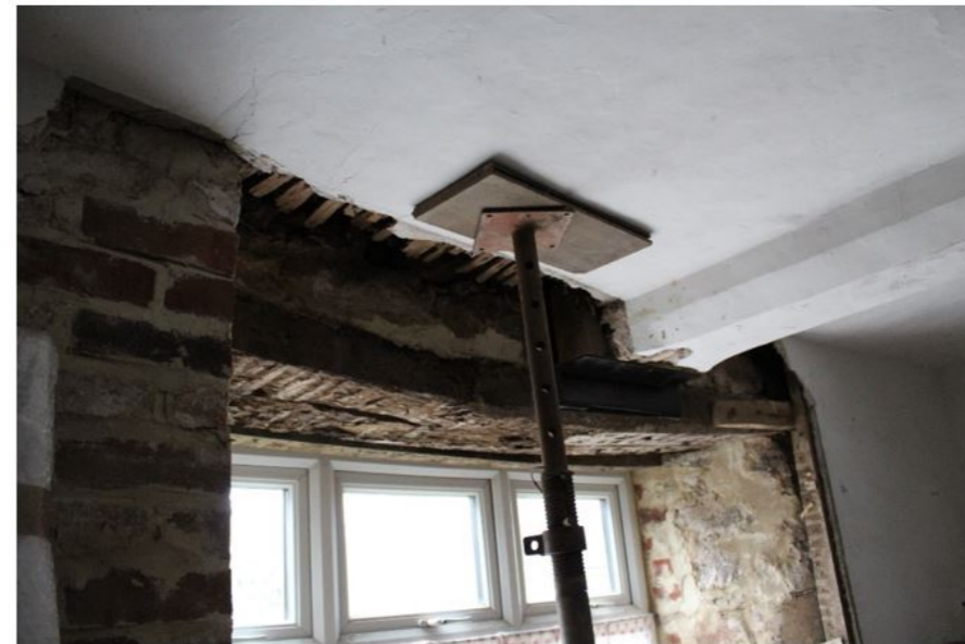
Fig. 7 Repair of beams and temporary propping of floor
