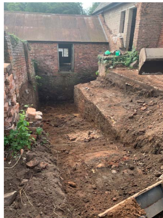
Earth Removal from Rear (AFTER)
