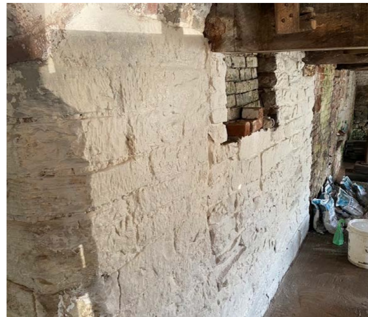
Internal walls being repointed and limewashed
