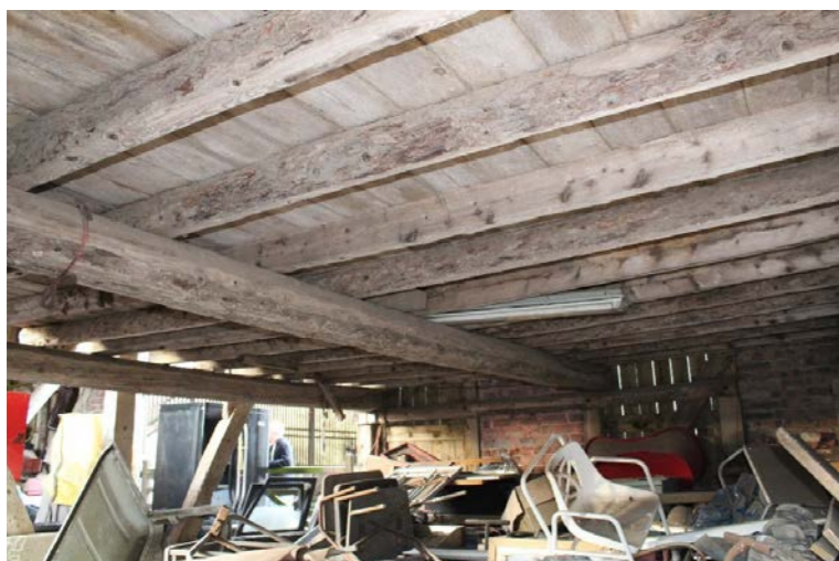
Fig. 7 Internal view to underside of first floor
