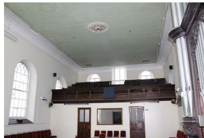
Fig.12 Internal view of Nave - has been recently repainted
