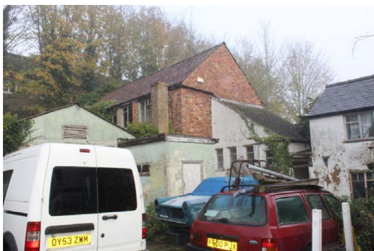
Fig. 7 Curtilage listed printing works and various 20th century outbuildings at rear are in poor condition
