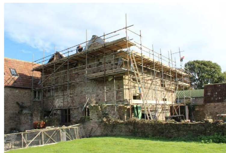
Fig. 20 Granary - Side and Rear Elevation
