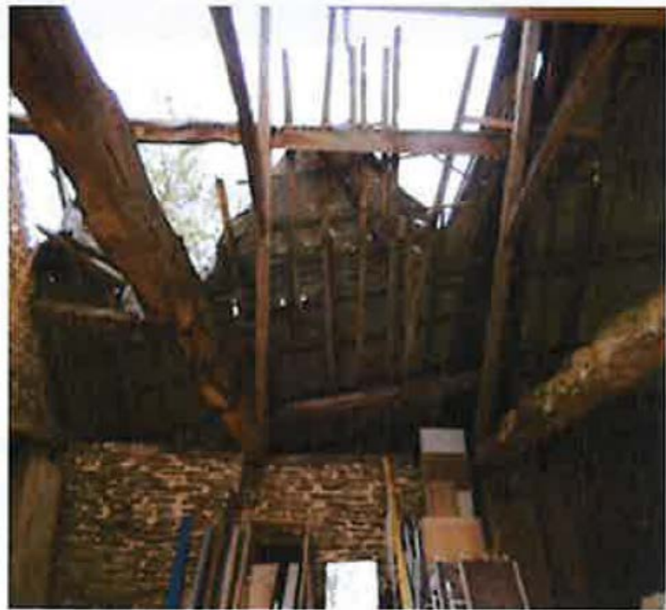
North Barn and Cart Shed 2017 Roof
