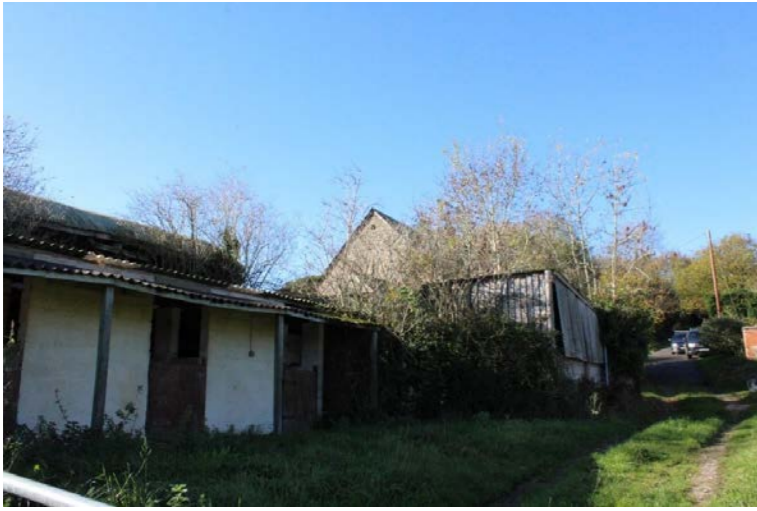
Fig. 3 Part side elevation (in background) is in fair condition
