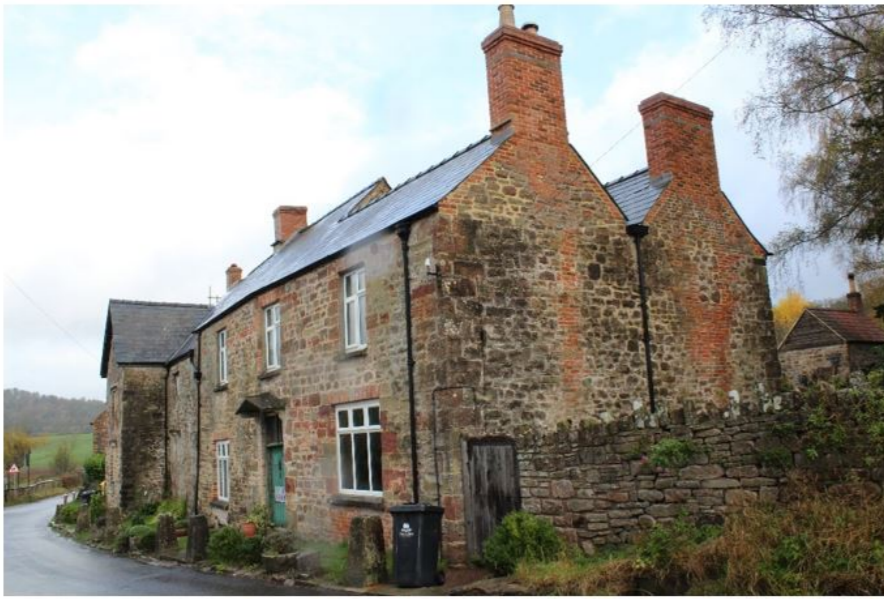
Fig.4 Front elevation - Spout Farmhouse in foreground
