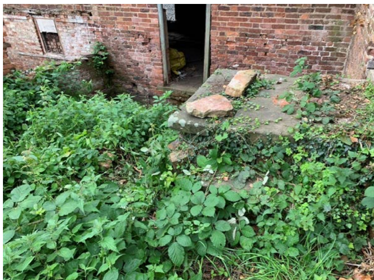
Earth Removal from Rear (BEFORE)
