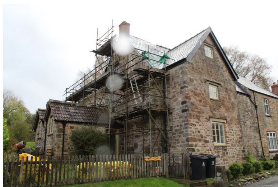
Fig.2 Front elevation - 1 Spout Cottage in foreground
