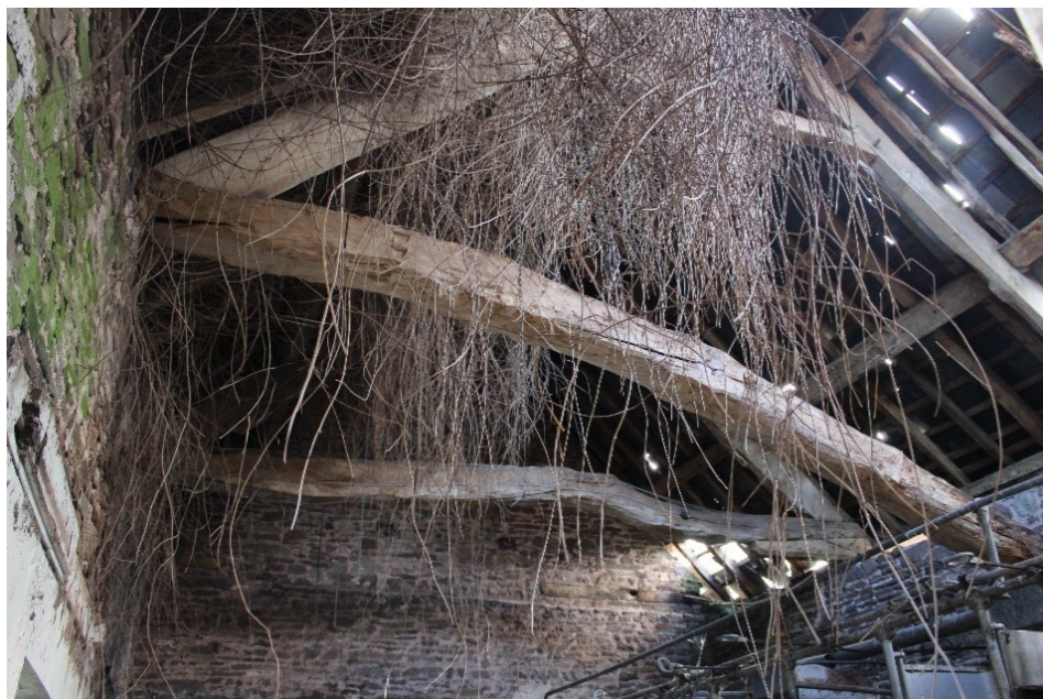
Fig. 12 Internal View - Roof and Walls
