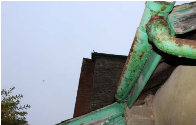
Fig. 9 Cast iron rain water goods
