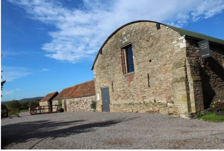
Fig. 15 South Cart Shed - Rear Elevation
