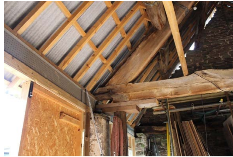
Fig. 10 North Barn and Cart Shed - Internal View
