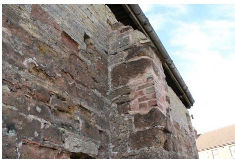
Fig.9 Modern repair to buttress
