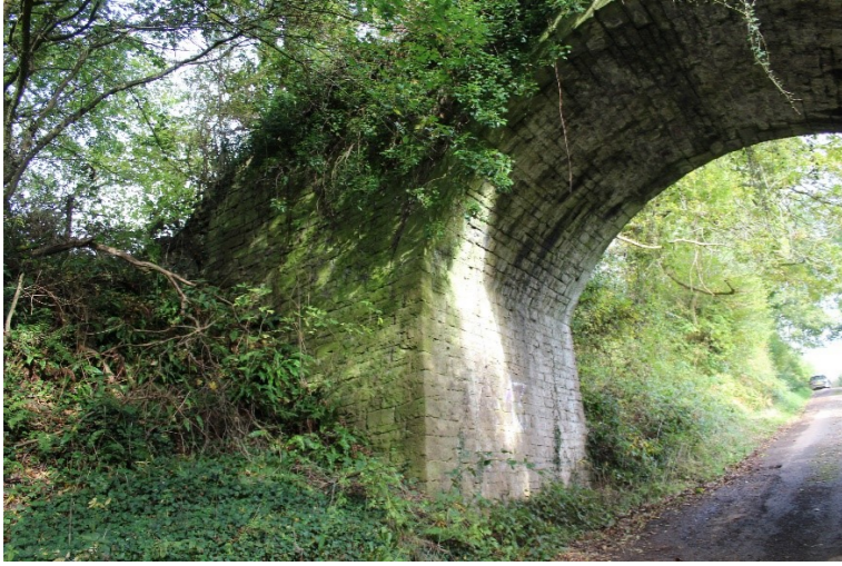
Fig. 3 Part elevation taken from lower road
