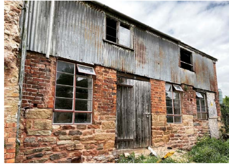
External wall AFTER removal of ivy and repointing work
