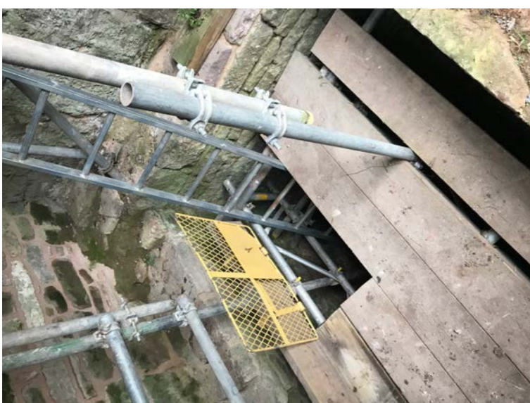
Fig. 3 Ladder access to wheel pit floor
