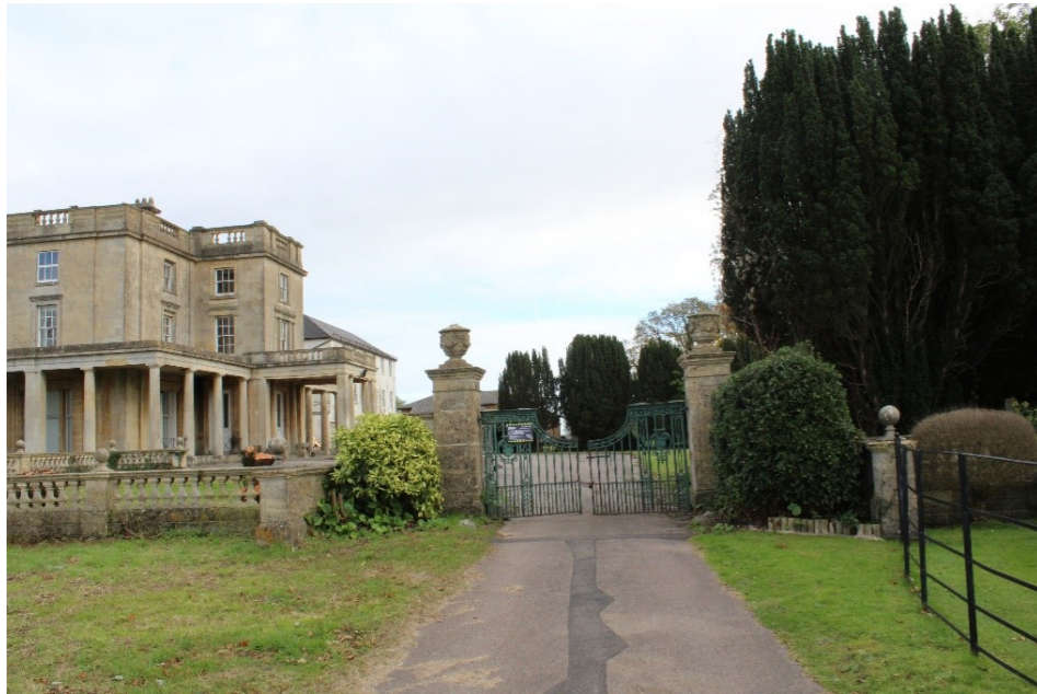
Fig. 1 Entrance gates locked but easily accessible
