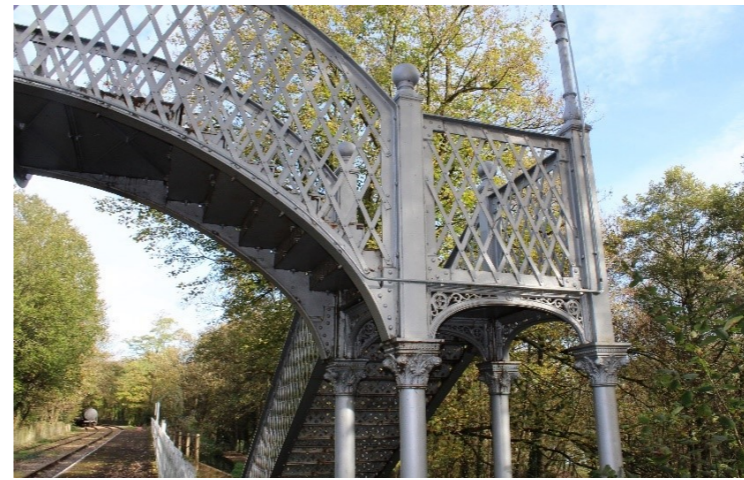
Fig.2 Stair and landing connecting to main span
