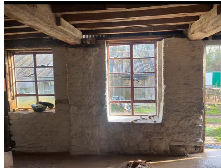
Internal wall AFTER repointing and limewashing
