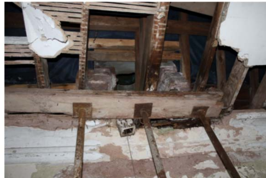
Fig. 14 Temporary propping of main ceiling structure
