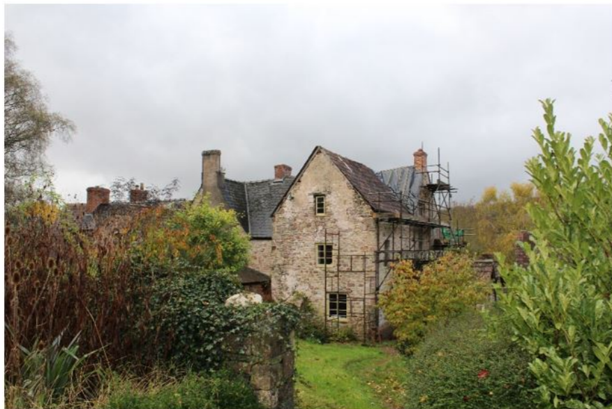
Fig. 6 Rear elevation - 1 Spout Cottage in foreground
