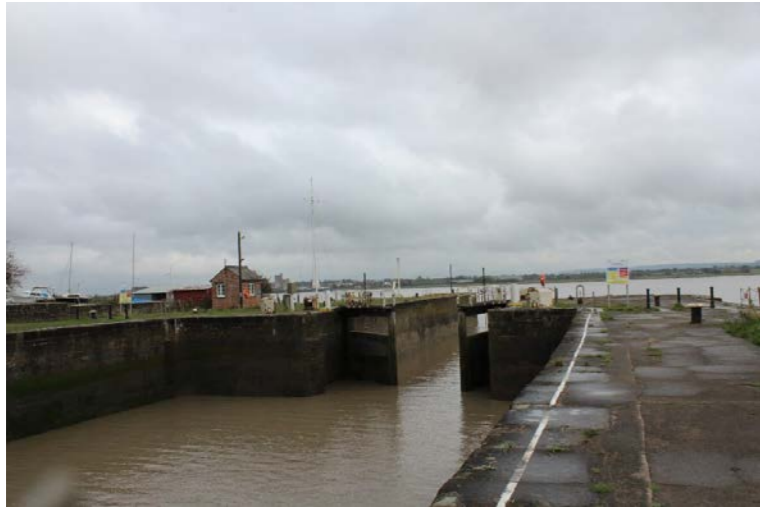
Fig.1 North and south pier and lock gate require repair. Harbourmasters building (on left) has been restored.
