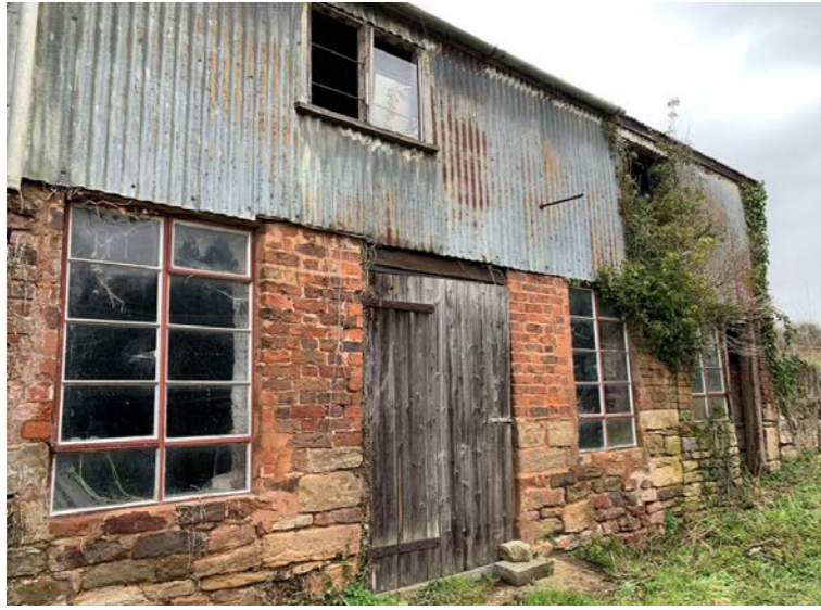
External wall BEFORE
