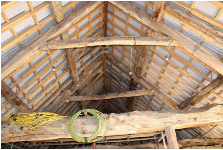
Fig. 9 North Barn and Cart Shed - Internal View
