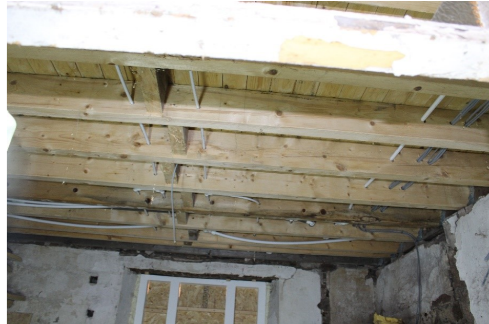
Fig. 6 Internal View - Upper Floor Repair/Replacement
