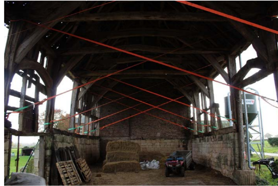
Fig.4 Temporary strapping restraining frame and preventing collapse.
