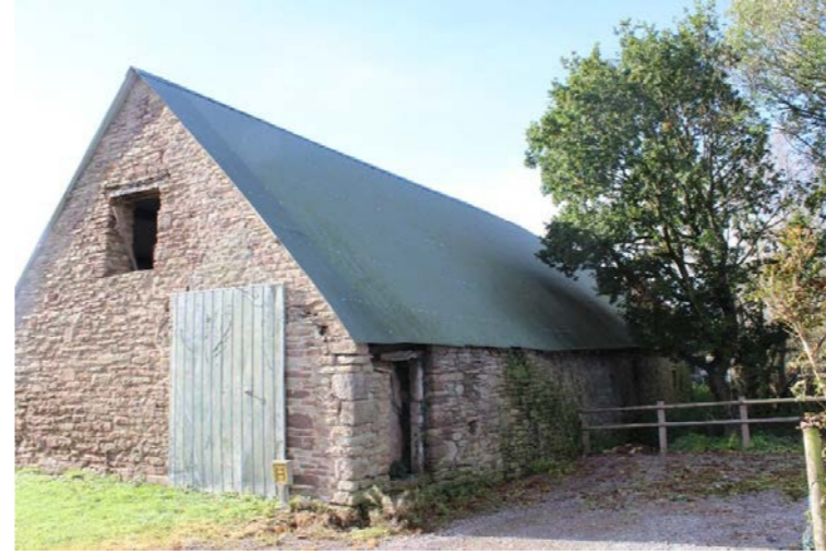
Fig. 8 North Barn and Cart Shed - Side and Rear Elevation
