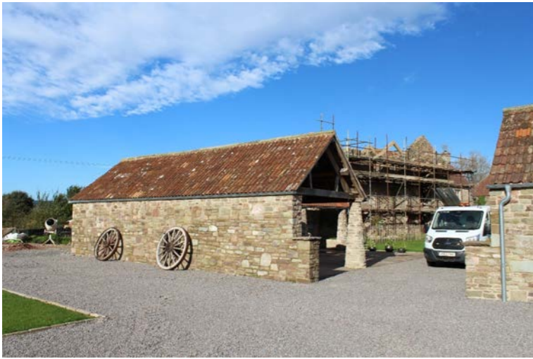
Fig. 17 Cart Shed - Side and Rear Elevation
