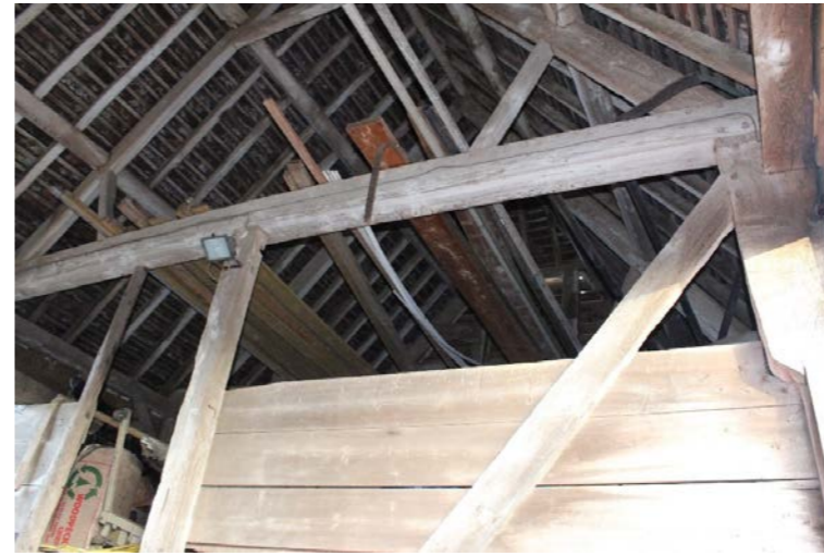
Fig. 6 Internal view of roof
