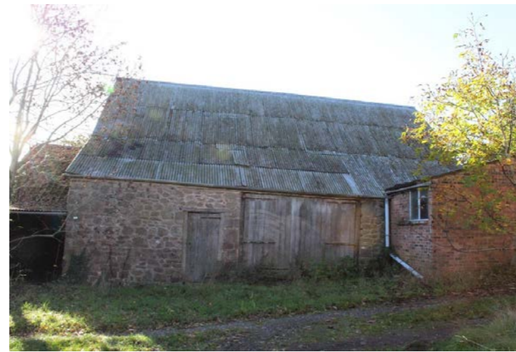
Fig. 2 Rear elevation - is in fair condition
