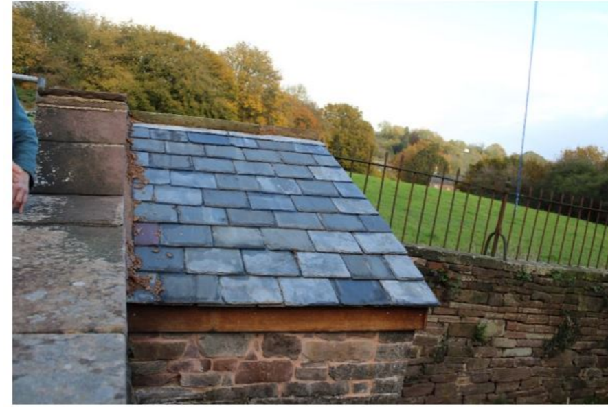
Fig.6 Toilet roof retiled
