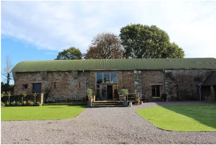
Fig. 11 Main Barn - Front Elevation
