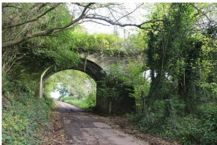
Fig.1 Part elevation taken from lower road
