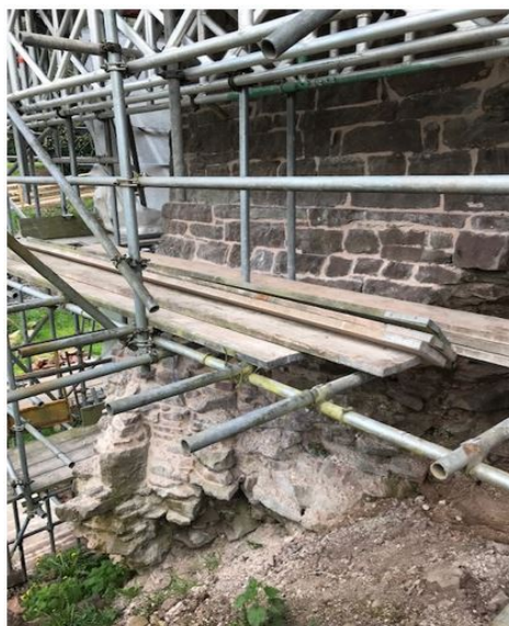
Fig. 1 Consolidation of the north wall
