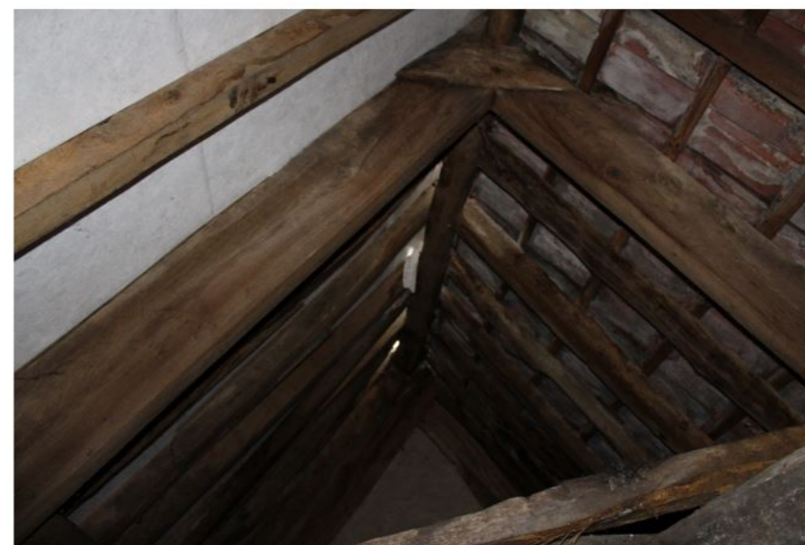
Fig. 9 Repair of roof in progress
