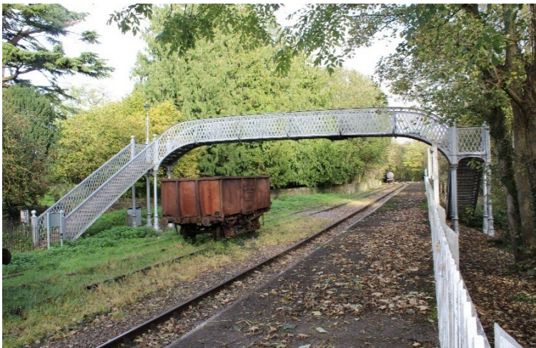
Fig. 1 Elevation of complete bridge
