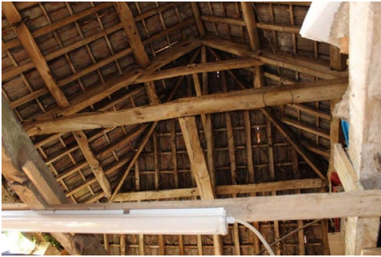
Fig. 5 Millhouse - Internal View of Roof Structure
