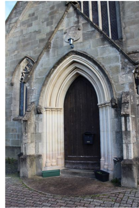
Fig. 2 Stonework to front door rebuilt
