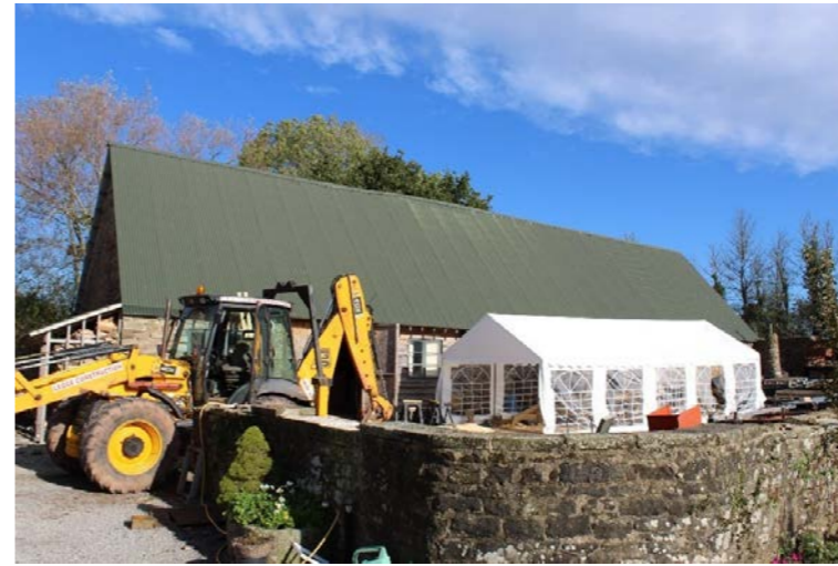
Fig. 6 North Barn and Cart Shed - Front Elevation
