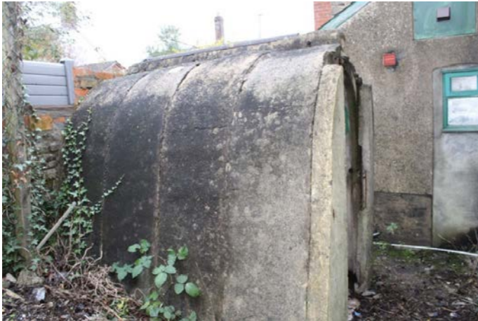
Fig. 7 Curtilage listed WWII Anderson shelter
