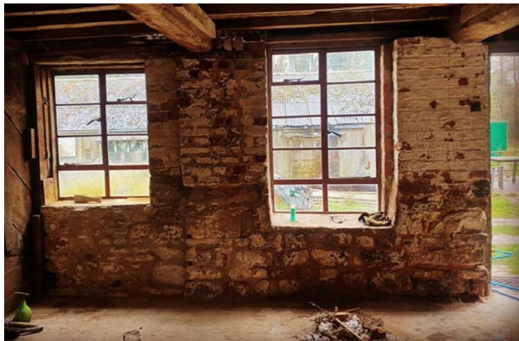
Internal wall BEFORE
