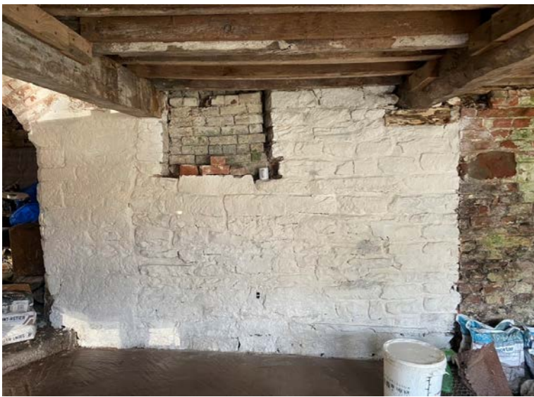
Internal walls (AFTER drying out) and being re-pointed and limewashed
