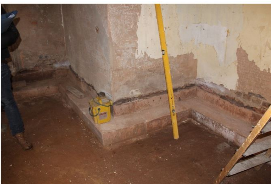
Fig. 10 Underpinning to stabilise walls in progress
