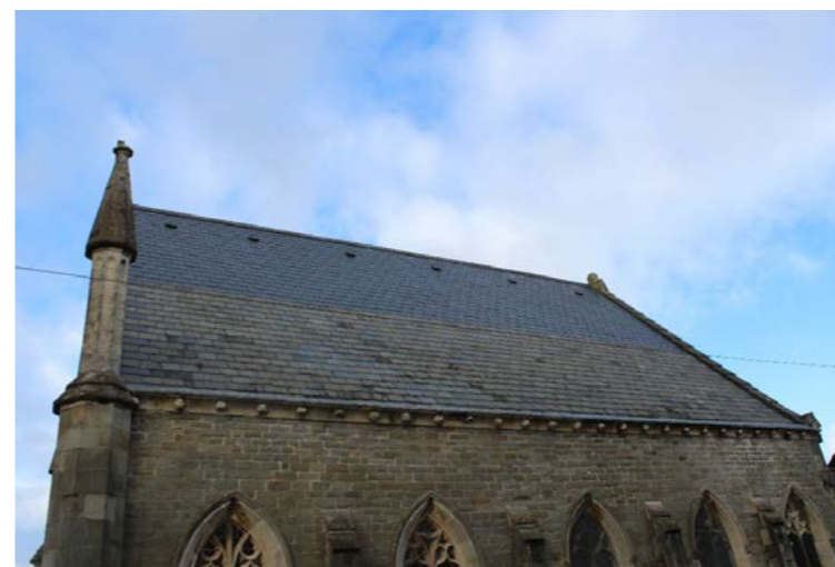
Fig. 6 Side and roof elevation
