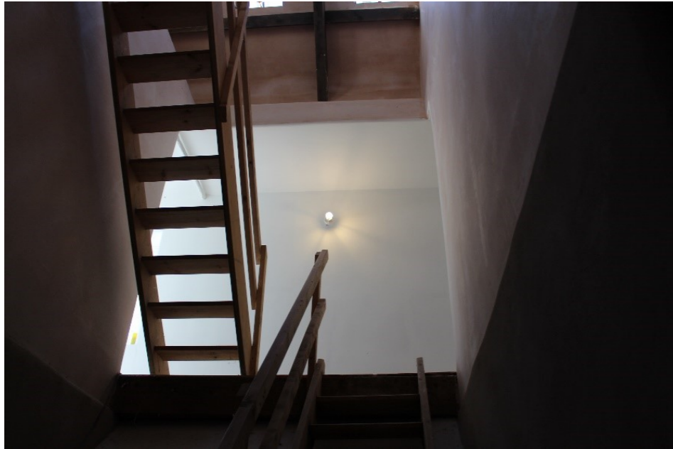
Fig.5 Internal View - Stairwell
