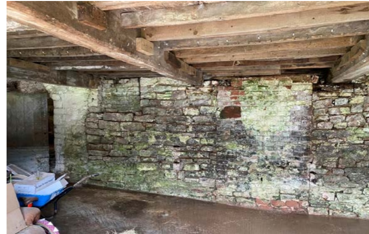
Internal walls (DURING drying out period)
