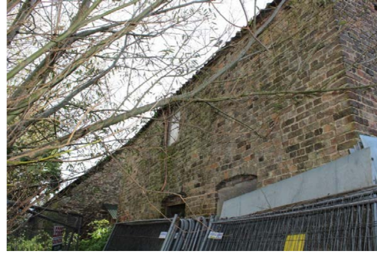
Fig. 4 Millhouse - Rear Elevation
