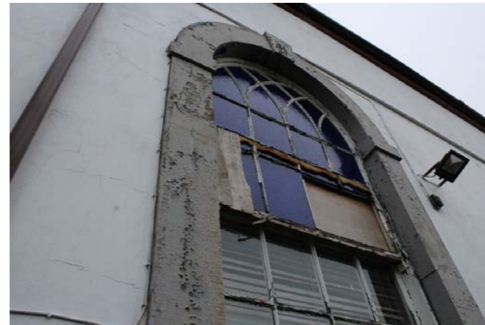
Fig.10 Nave timber window frames
