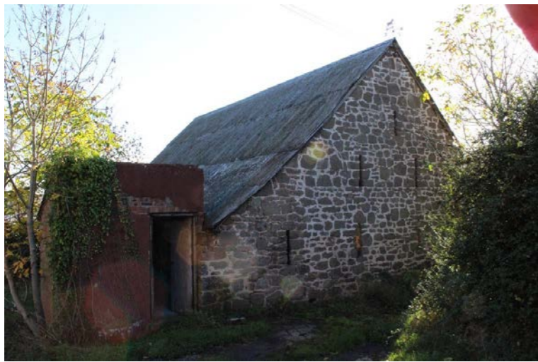
Fig. 1 Side elevation - is in fair condition
