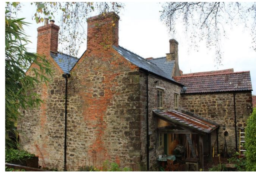
Fig. 5 Side elevation - Spout Farmhouse in foreground
