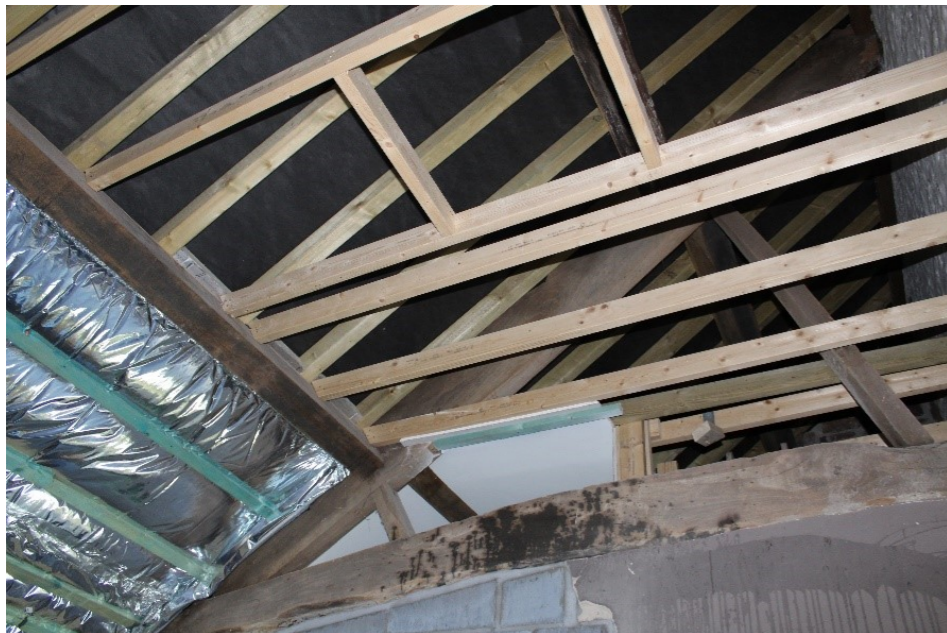
Fig.7 Internal View - Roof Repair/Replacement
