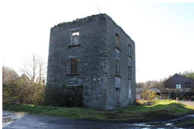
Fig. 3 Rear elevation in foreground
