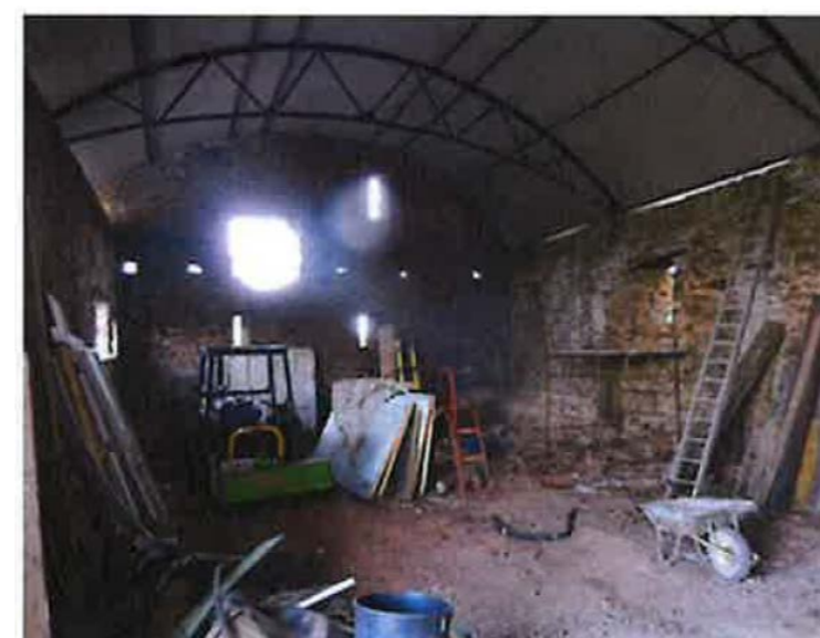
Inside Main Barn repairs 2017
