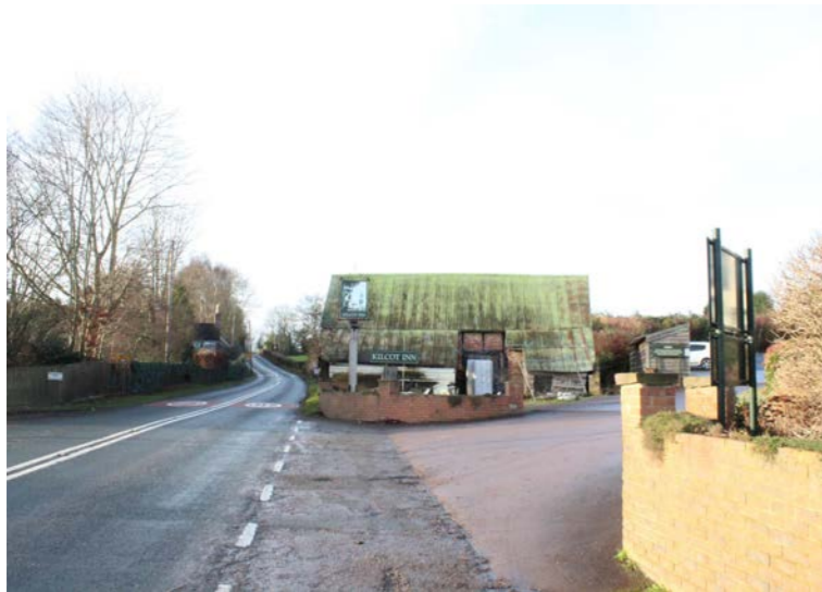
Fig.1 Front elevation - in poor condition
