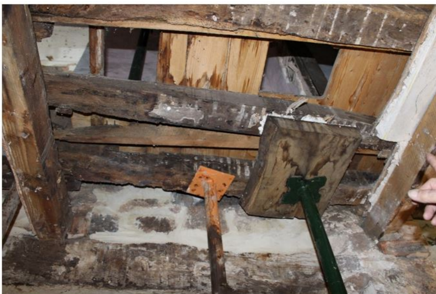
Fig. 8 Repair of beams and temporary propping of floor
