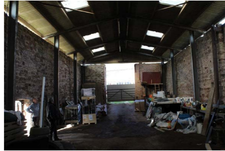
Fig. 4 Internal view towards front elevation
