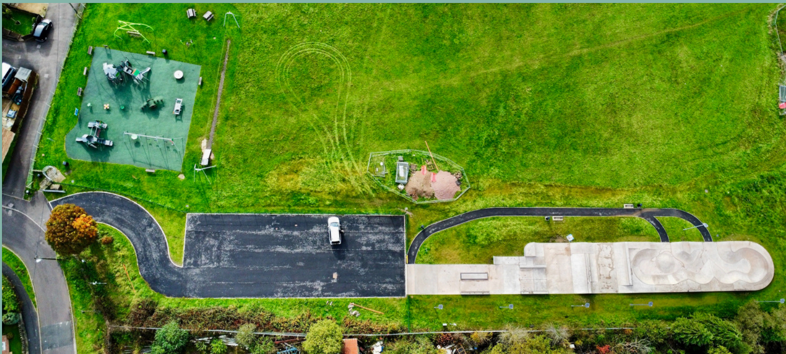
Aerial view of Cinderford new skate park
