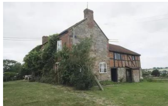
Gamage Hall, Dymock. Grade II. List Entry 1341940
