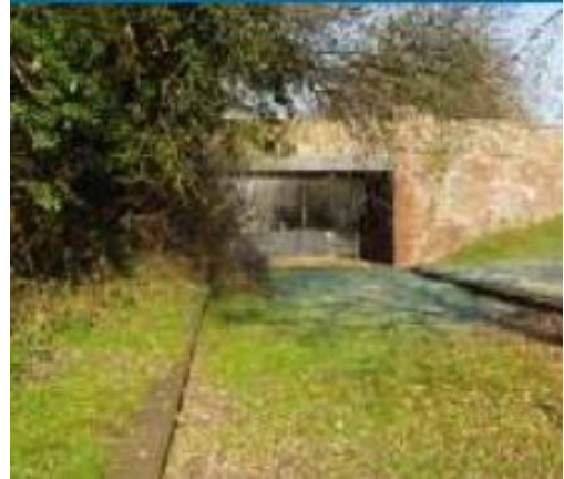
Restored road bridge by Western Way
