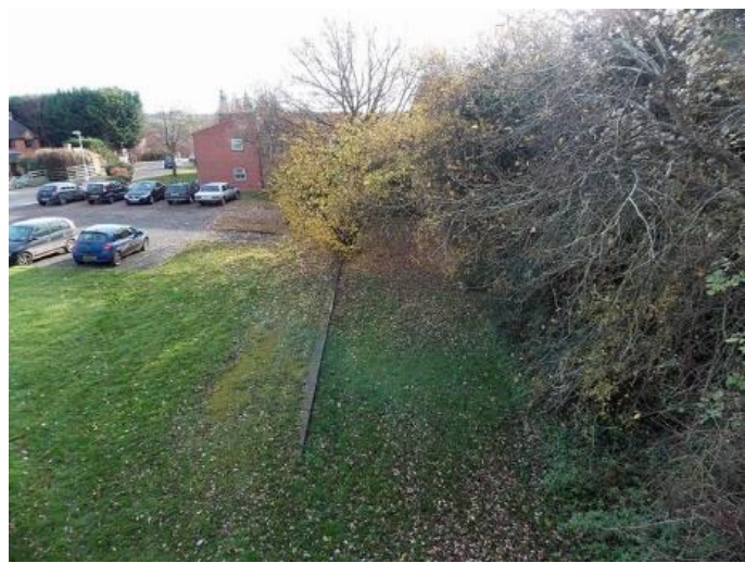
Remains of the station platform visible in Western Way
