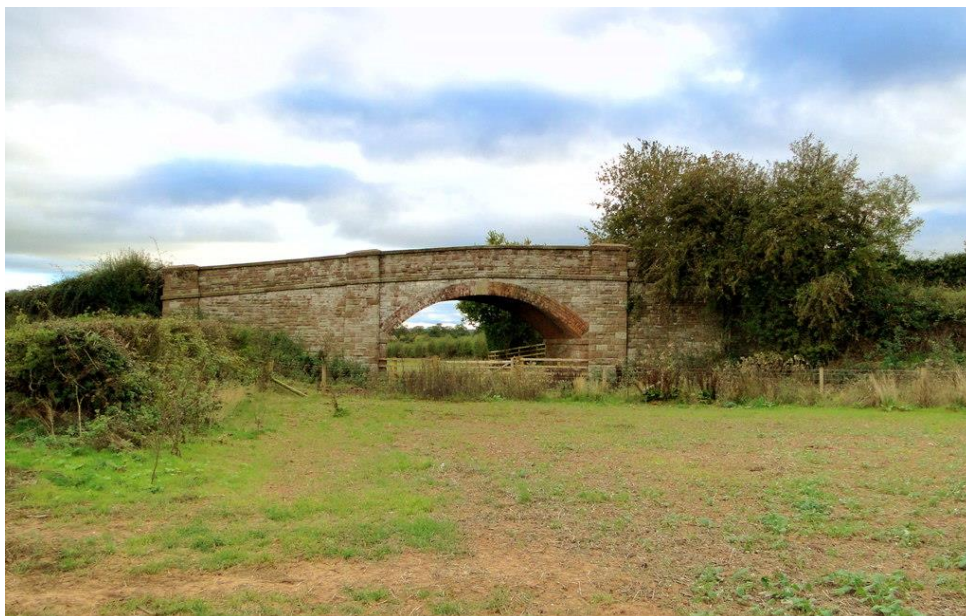
Former railway bridge at Tiller's Green
