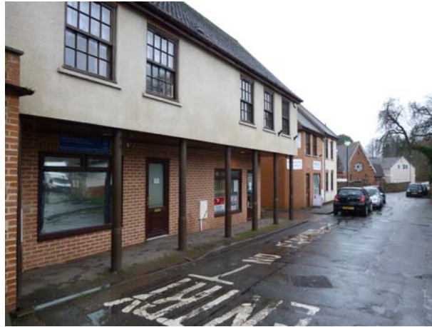
Figure 90 - Howell Jones Building, Court Lane
