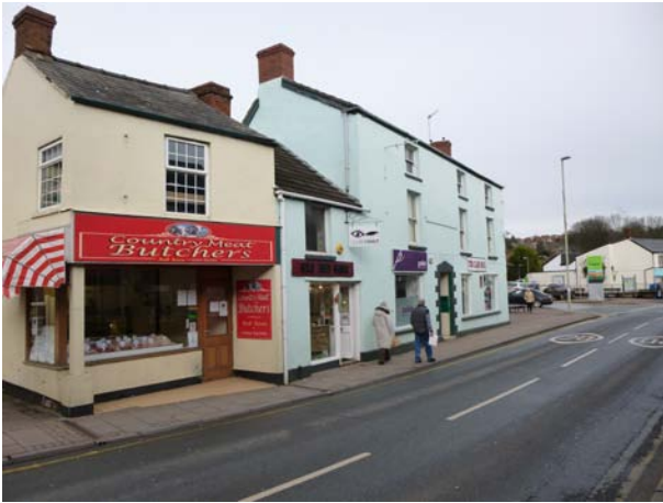
Figure 68 - Northern side of Newerne Street
