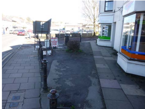
Figure 103 - Area in front of Bridge House, Newerne Street
