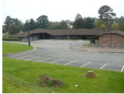
34 Pyart Court below the road level, with
