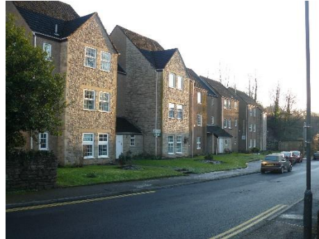
H11 Pavements and layby at Marine Gardens. In summer residents gather around a table on the open plan frontage, which increases feeling of community.
