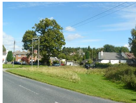
52 The view of the oak is somewhat marred by the electricity transformer. The meend has been part mown and the paddock is to the right. A valuable green space.
