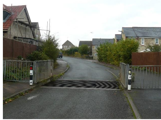
SA19 Cattle grid to prevent the Forest sheep entering Primrose Drive estate
