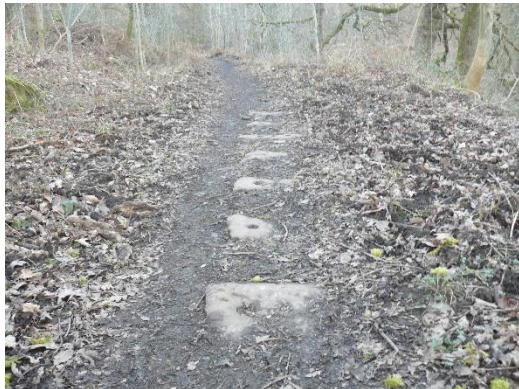
GRS9. Tram Road, showing stone settings for the rails
