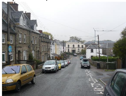
A2 On-street parking both sides of the one-way street up to the (closed) church detracts from older buildings
