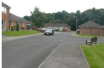
F5 the mature trees along the cycle track can be seen in the background, and a parking court is off to the right of the picture.
