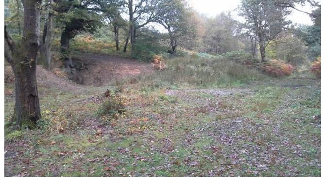
GRS8. Entrance to coal level, centre left, now disused and made safe
