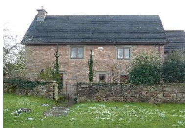
27 Scowles Farm with its carved pediment and stone mullion windows. These are unusual, given the, irregular, not dressed, stones. The slate roof and chimney look newer.
