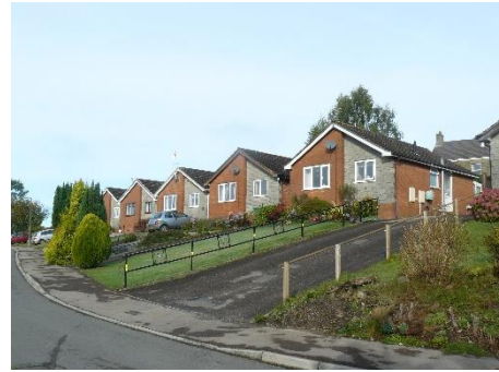
C6 Bungalows in Lark Rise almost at the brow of Sunnybank
