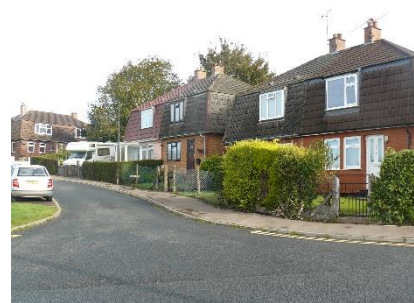
C4 Cornish Houses along the green with layby parking, and some on plot taken out of front gardens
