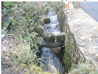
10. Culvert collapse (since repaired) near to the quarry entrance.
