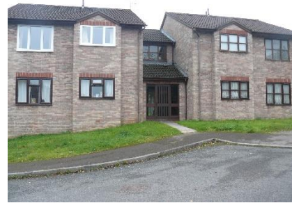
F14 Blocks of 1 and 2 bed flats with parking courts, some of which are surfaced with pavers
