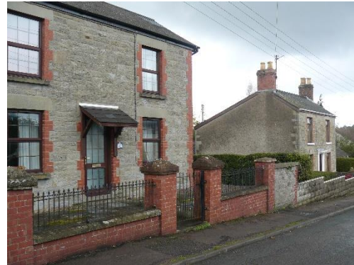
SA10. Use of local stone and brick in 19C construction, with chimneys as local coal was used for fires; larger back than front gardens to provide for vegetable plots.
