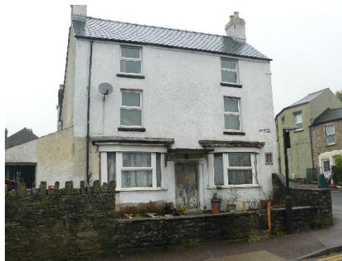
A12 Originally the Mason's Arms Pub, now residential, but in a key position on the way into town from Monmouth
