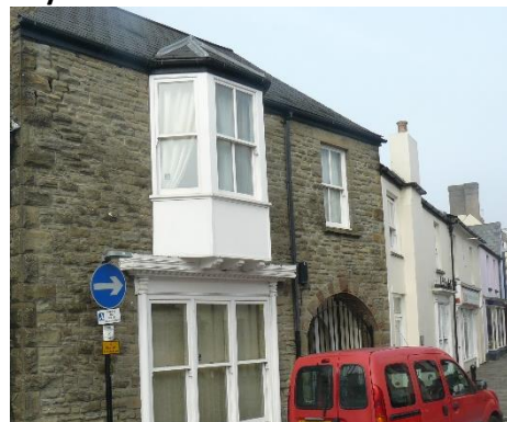
21 Old Wine Vaults – now Housing Association
