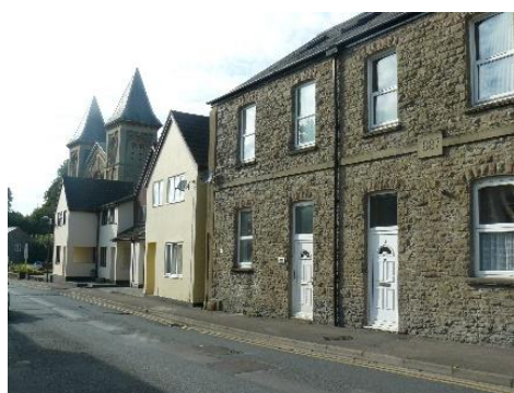
H7 The British Schoolroom was converted into housing along with the modern infill shown, to give a varried streetscape, maintaining the exterior of dressed Forest stone from 1887 and sash style
