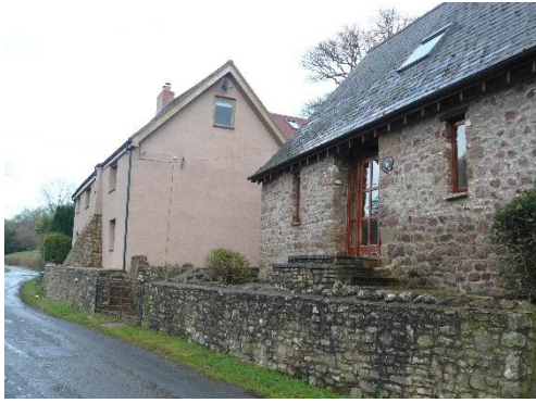
16 Older possibly medieval house to the rear, with buttresses, raised floor above the flood level, and a barn conversion
