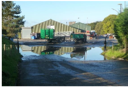
42 Concrete Utilities manufactures large concrete products eg streetlights which require heavy transport, so is sited off this main route.
