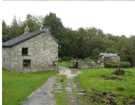
4. This local stone shows keys which are irregular, and differently sized blocks, possibly built by a quarryman for their family. The forest shed on the right and the
