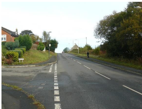
11. Looking back to the brow of the hill, with the entrance to the Hospice on the right behind the hedge
