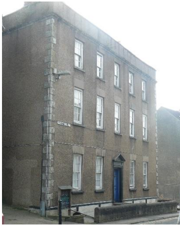
H16 Caragh House Flats 3 storeys with a basement and parapet roof and once the home of James Teague, this is now flats. The pebble-dash does not cover the keystones on the corners, where evidence of the fixings to the original iron railings is still present. The front door with its architrave and pediment is a classic Georgian feature. The building is in need of some maintenance, using skills and materials appropriate for its listed status.
