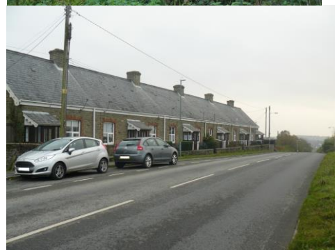
10. The Gorse Almshouses, with small layby, built of stone and slate with classic porches and short chimneys
