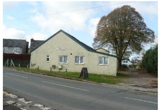
24 Evergreen Hall – 3 community buildings within 50 yards of each other
