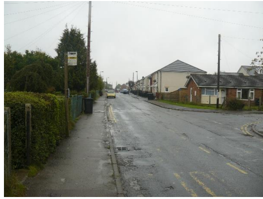
SA4 Note the straight linear look of housing and the poor condition of Tufthorn Ave near the junction with Stepbridge Road, the industrial area. The bungalows, right, are for older people
