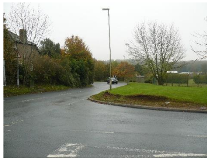
80 Suntory is the turning right, and the car is approaching from the traffic lights around the sharp bend. HGVs have to proceed slowly in the centre of the road.
