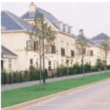
The choice of materials and design of boundary features should pay due regard to local character.
