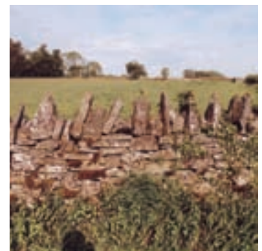
Boundary wall sometimes have distinctive copings such as this 'cock and hen' cope.
