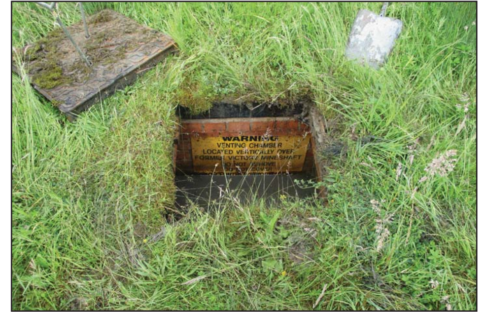
Victory Mine venting chamber, looking west
