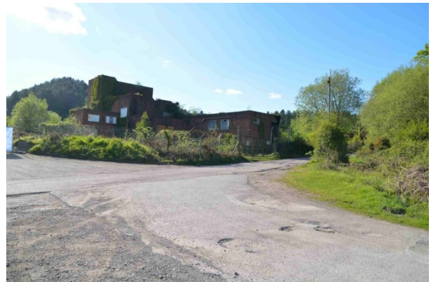
Photograph 2: Survey Corridor 2, from the east
