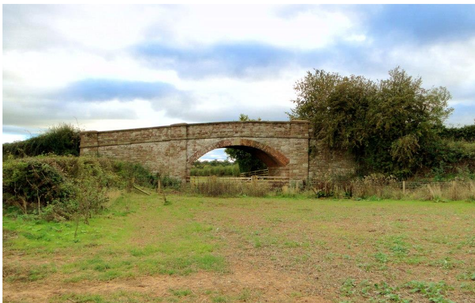
Former railway bridge at Tiller's Green
