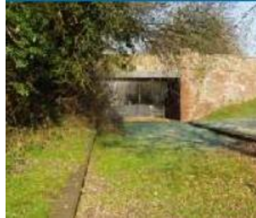
Restored road bridge by Western Way
