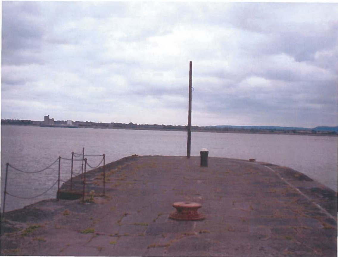
4. Views from lock gates across estuary
