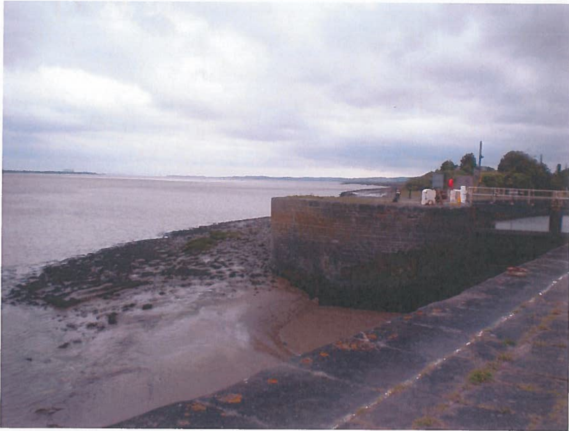
5. View south from lock gates to the Severn Crossings about 20km distant
