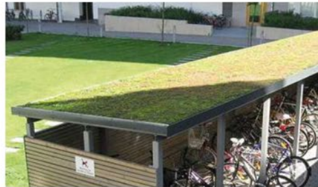
Green sedum roof to cycle shelter
