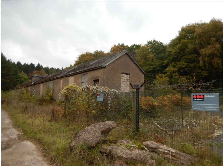
South and Western Elevation (From South)
