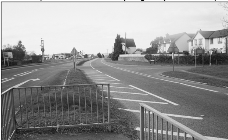
The A48 Village Junction – a major hazard
