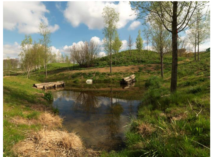
Figure 9-16 – SuDS pond showing inlet on far bank
