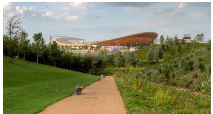
Figure 9-7 – Swale construction on the London 2012 Olympic Park (before and after)
