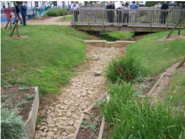
Figure 10-9 – Slot weirs
