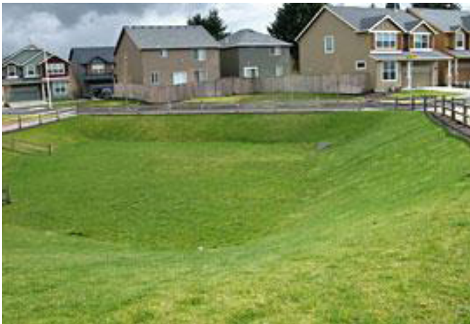
Figure 9-19 – Detention pond - empty
