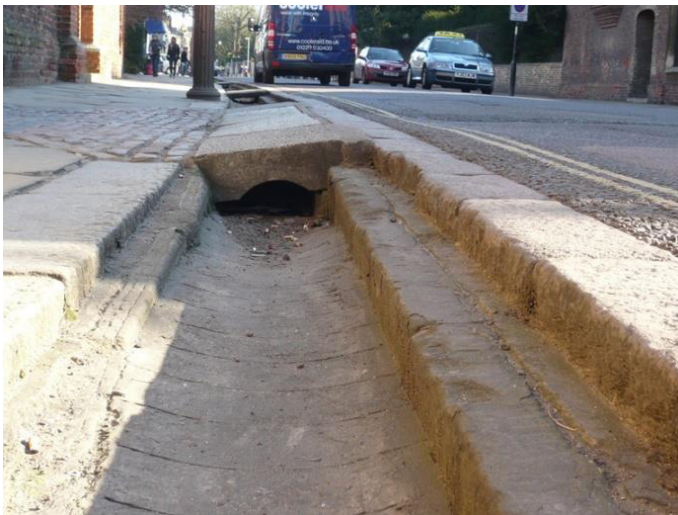
Figure 9-44 – Typical SuDS channel
