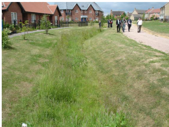
Figure 9-4 – Dry swale during rainfall showing gully outlet (SuDSnet)
