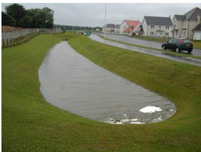
Figure 9-21 – Detention pond - full
