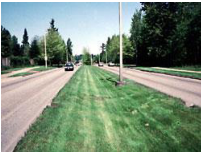
Figure 7-1 – Examples of source control including, swales, permeable paving, bioretention and green roofs (clockwise from top left)
