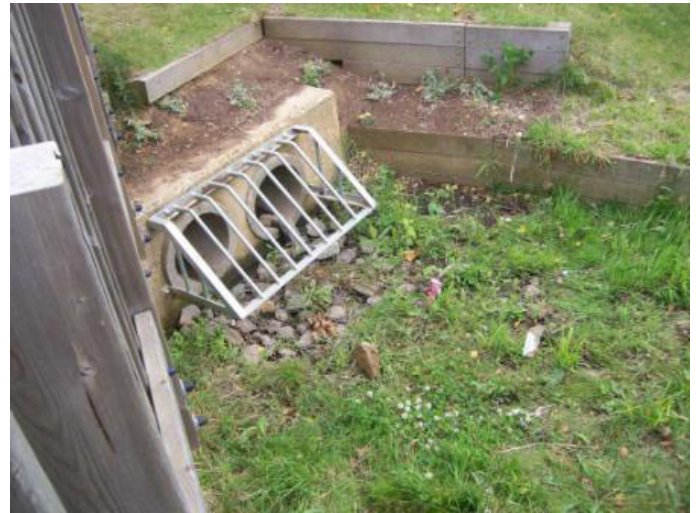
Figure 10-5 – SuDS outlet with trash screen
