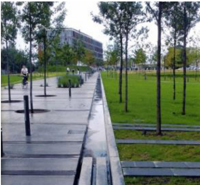
Figure 9-40 – Typical rill channel (Susdrain)
