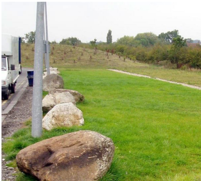
Figure 9-8 - Grass filter strip at the edge of a parking area (Susdrain)
