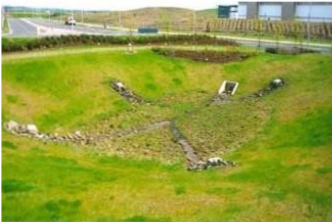
Figure 10-1 – SuDS pond with inlets and outlet
