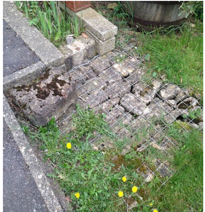
Figure 10-3 – Inlet and outlet using a stone basket
