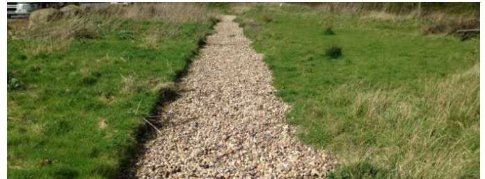
Figure 9 27 - Filter drain (SuDSwales)
