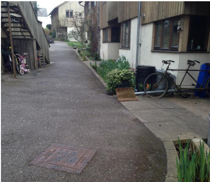
Figure 9-43 – Typical rill channel linked to downpipes
