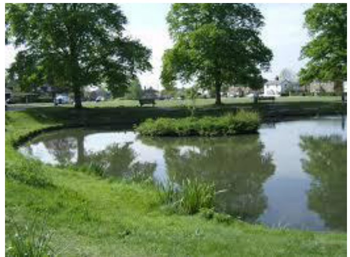
Figure 9-15 – Typical SuDS pond
