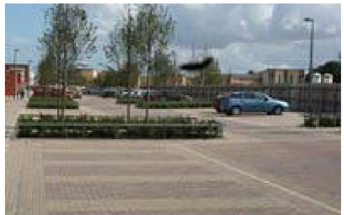
Figure 9-33 - Permeable pavement in a car park
