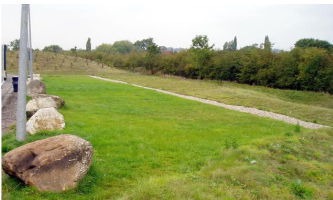
Figure 9 26 - Filter drain protected by grass filter strip (Susdrain)
