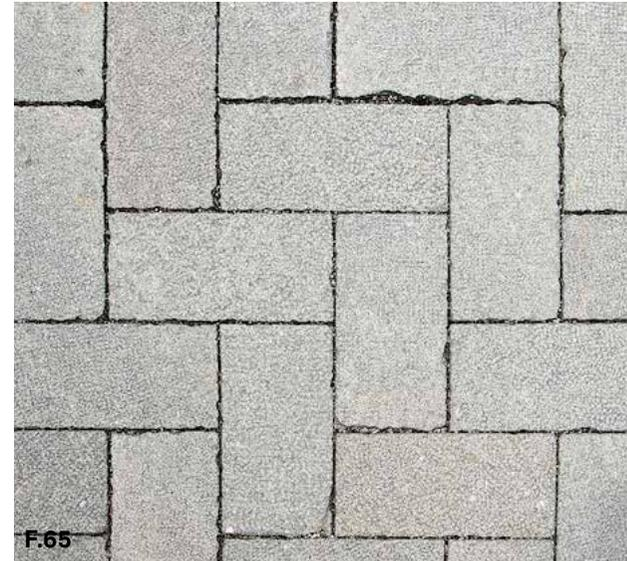
**Figure 65:** Permeable paving laid onto open graded bedding, base and subbase layers allow percolation of water into earth.
